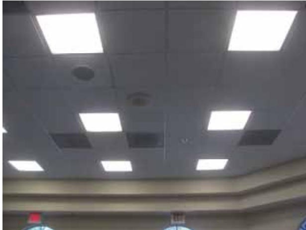
Acoustical ceiling tiles at exercise room
