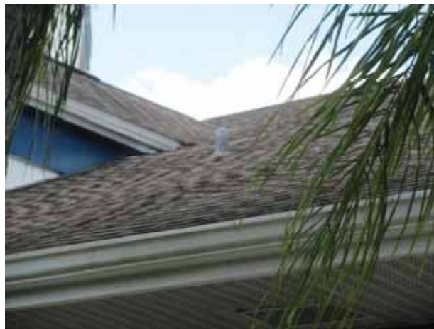
Asphalt shingle roof at clubhouse
