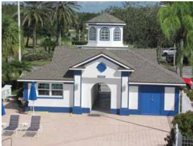
Pool cabana building
