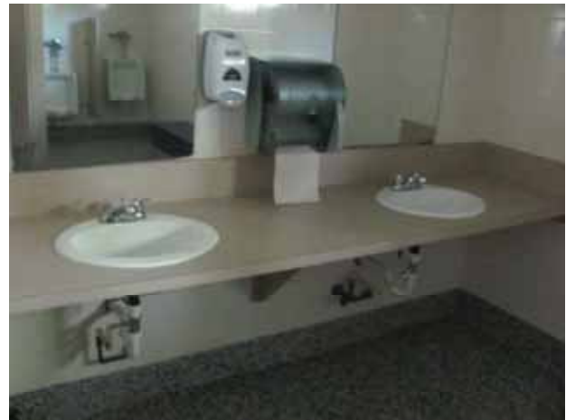
Pool cabana building
