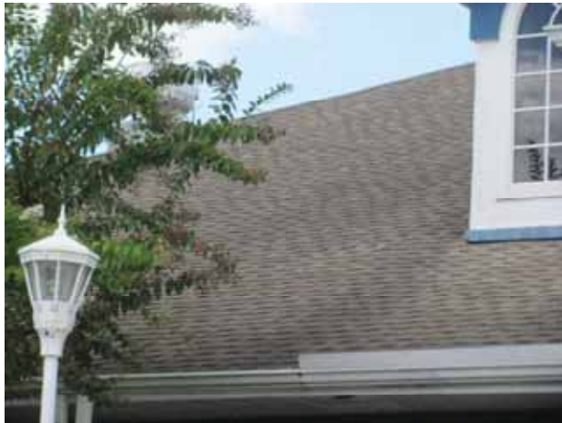
Asphalt shingle roof at clubhouse
