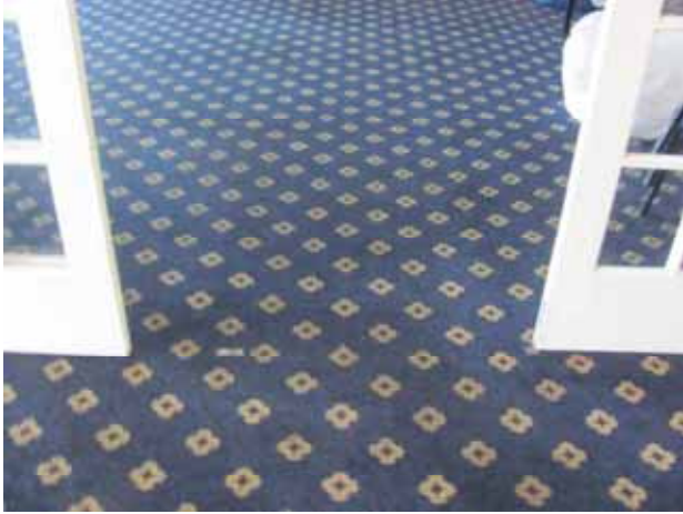
Carpet floor coverings at bay room
