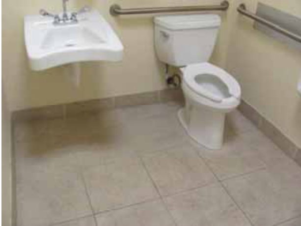
Ceramic tile floor coverings at rest room
