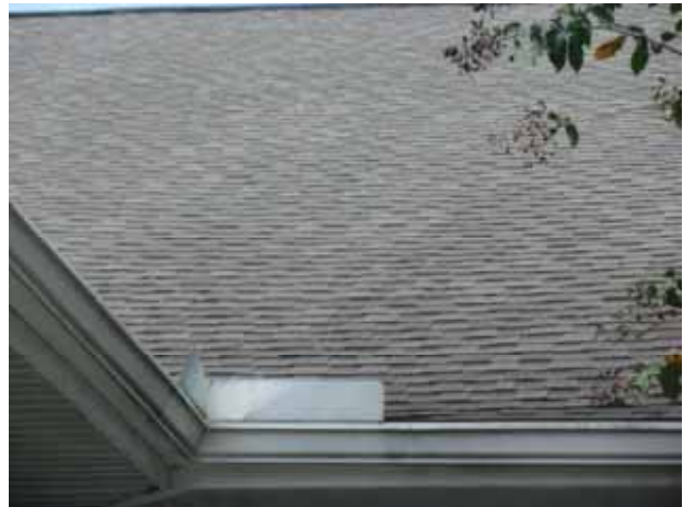
Asphalt shingle roof at clubhouse
